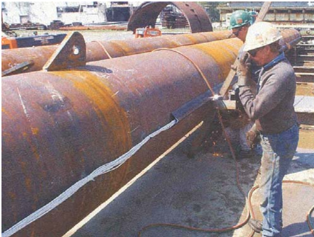
Installation of resistance strain gages on large diameter pipe pile foundation.
