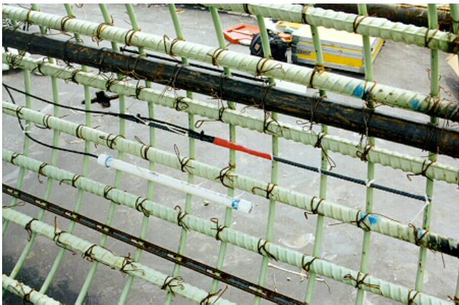
(below) Sisterbar resistance strain gage instrumentation for drilled shaft foundations.
