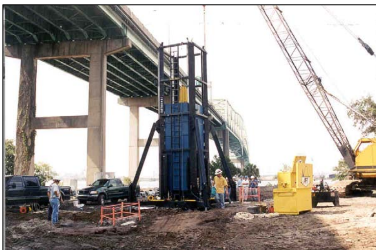
(Below) 500 ton Statnamic Load Test. (Mathews Bridge)
