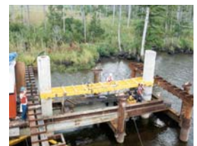
Lateral Static Load testing
