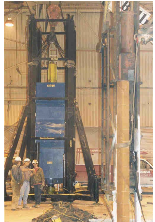
Catch mechanism STATNAMIC load test on pipe piles inside an automobile factory. Illinois
